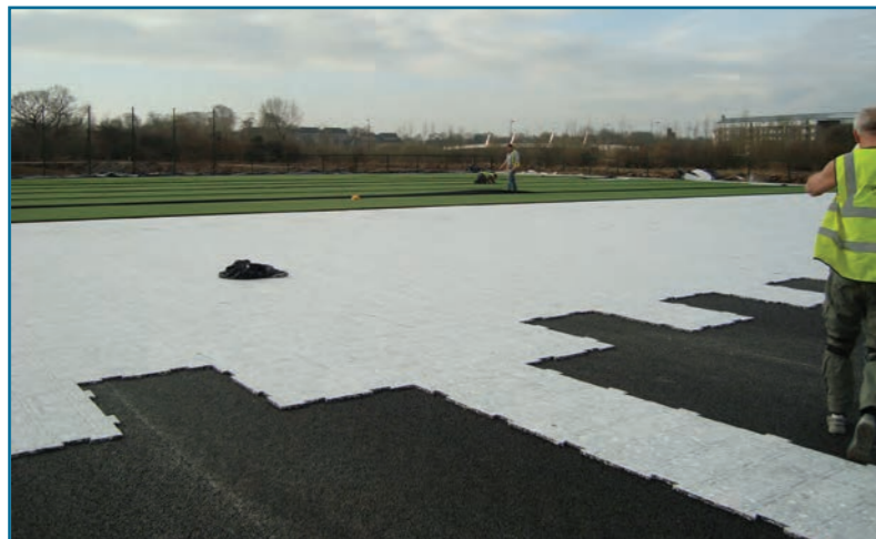
Figure 7 - Shockpad laid as tiles on an asphalt base
